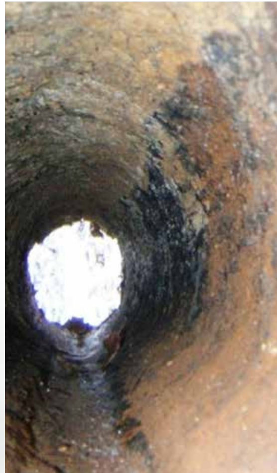
Figure 3: Pipe Invert Abrasion
