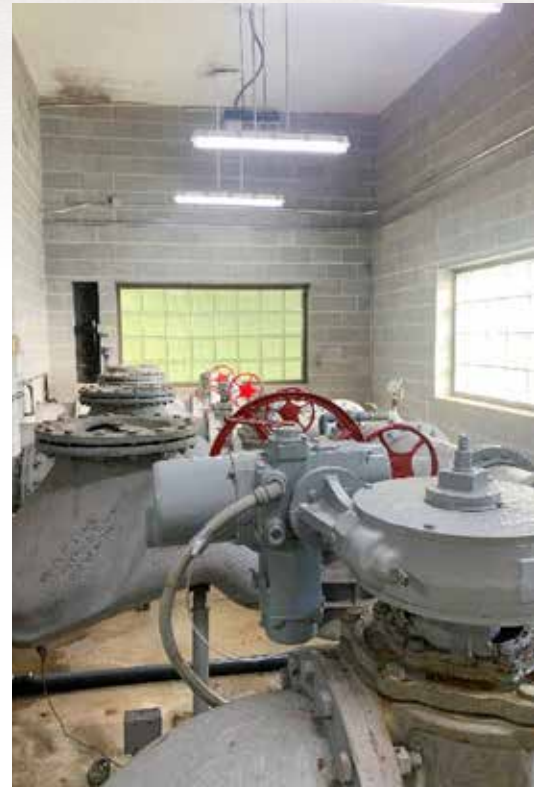
Figure 4: Lift Station Check Valves - Insertion Points
