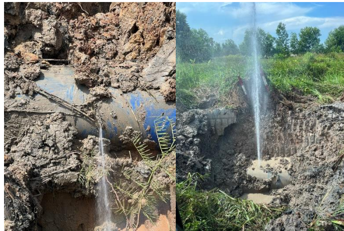
Figure 7: Pictures of two leaks located by the free-floating Pipers® and repaired by DTS at 8942 m (left) and 9001.8 m (right).
